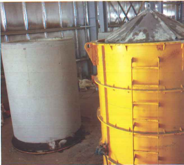
1 – A Pouring cone used to distribute fresh concrete into the forms
