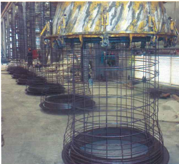
1- Outer mould picking up the pallet with reinforcement cage
