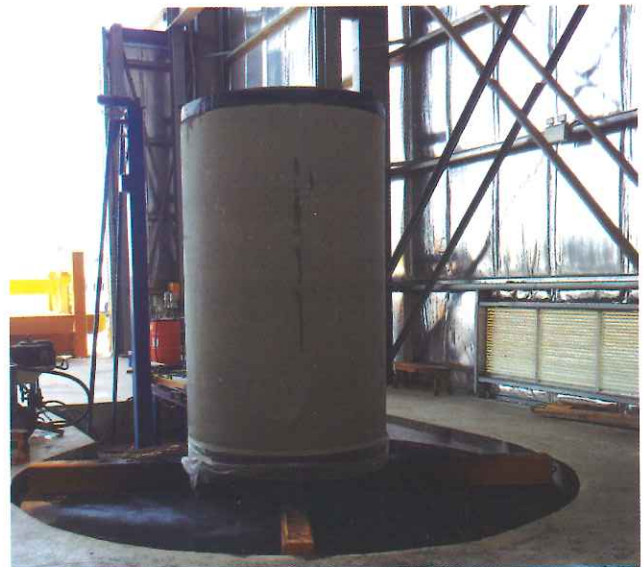
4 – Protective coating is being applied by airless spray
