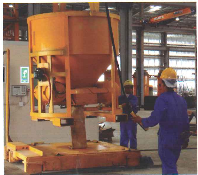
2 – Concrete is placed in the bucket and transported by crane
